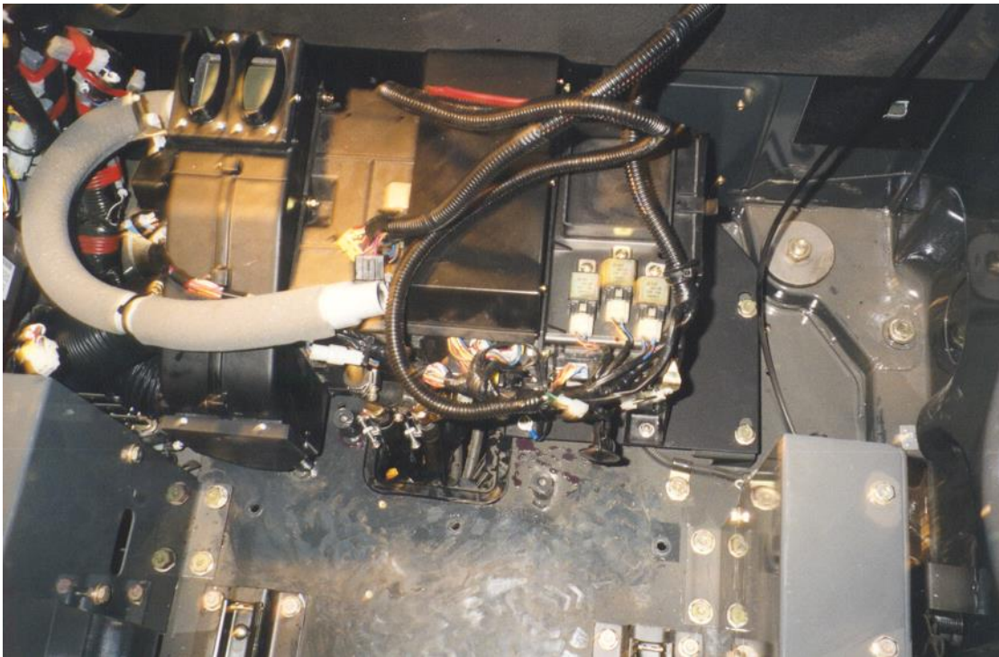
Evaporator assembly mounted in place.
